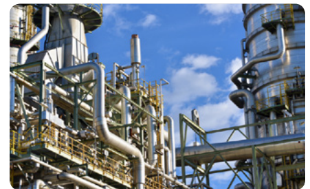
Kraftwerksbau | Power plant construction
